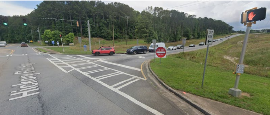
The SR 140 off-ramp design increases the potential for wrong-way drivers. Additional signage along SR 140 and up-stream of off ramps can help to deter wrong way drivers
