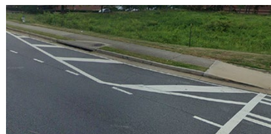
Painted bulb-outs that could be formalized with concrete
