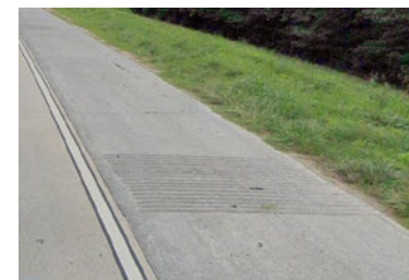
Rumble strips are spaced at nearly 50' apart along some segments of the corridor.
