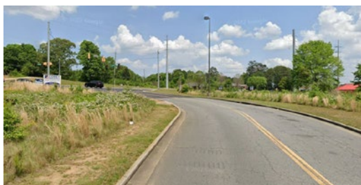
Limited sight distance on northbound Lovejoy Lane
