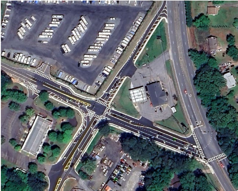
An intersection improvement project was recently completed that re-configured the intersection.
