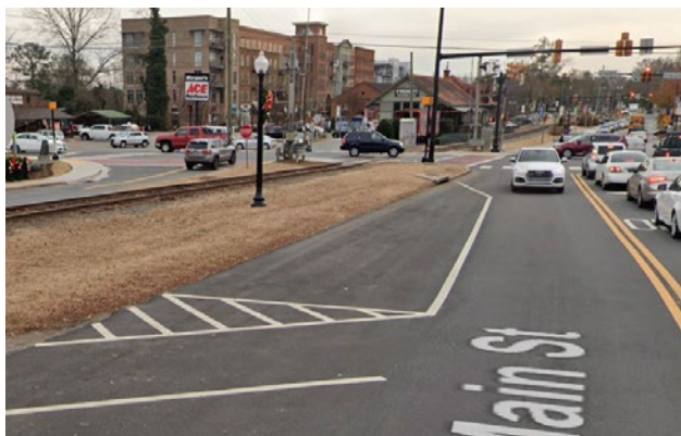
Excess space between the Arnold Mill Road signal and on-street parking could be land-scaped to slow traffic
