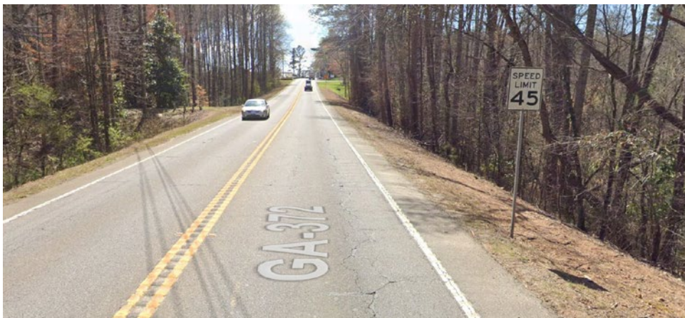
The corridor quickly transitions from a high speed rural roadway into Downtown Ball Ground
