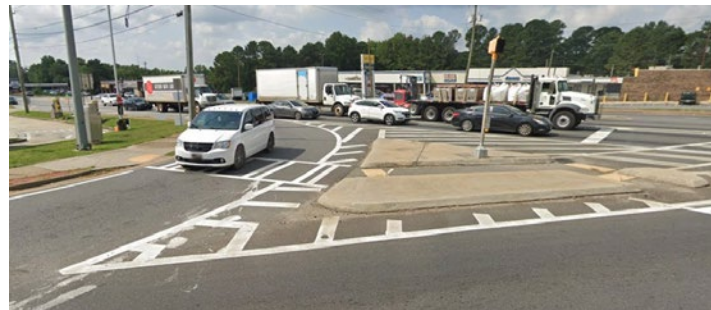
The design of the existing channelized-turn islands encourage sweeping right turns, and force drivers to look over their shoulders to see oncoming traffic
