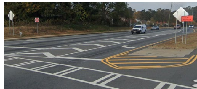
Median noses can be extended to provide pedestrian refuge
