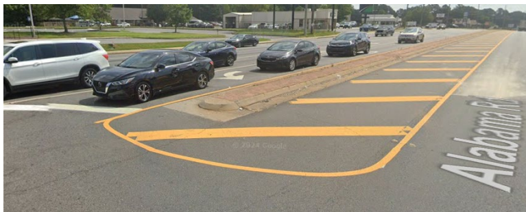
The mainline median noses are wide and could be extended into the crosswalk to provide pedestrian refuge
