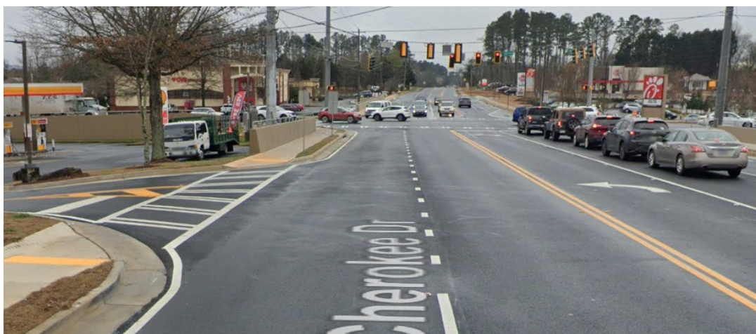
Vehicles can currently turn left into and out of the Shell Station drive-way location just south of the intersection, introducing additional intersection conflicts
