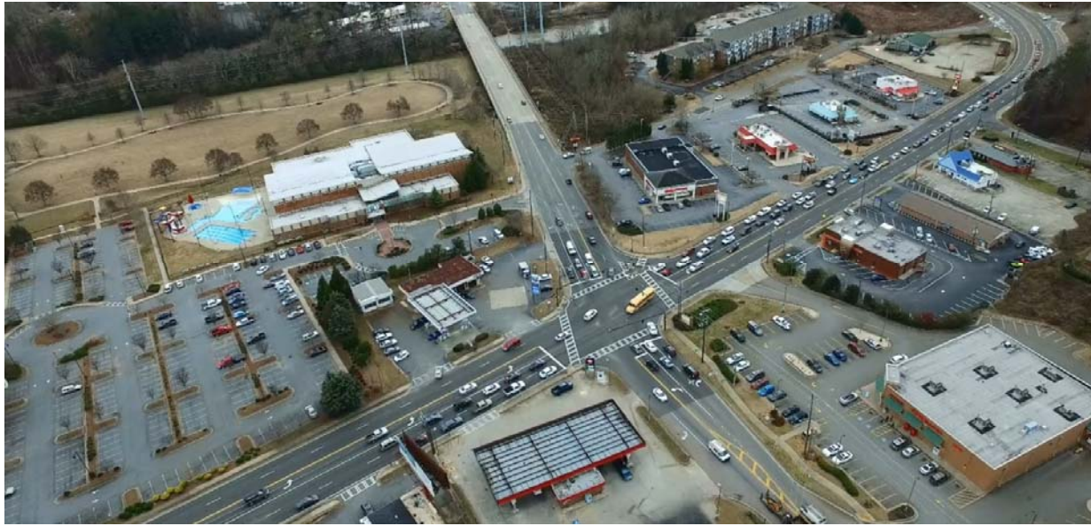
Figure 2-2 - Drone Image – SR 140 at Marietta Hwy/Riverstone Pkwy – AM Peak Period
