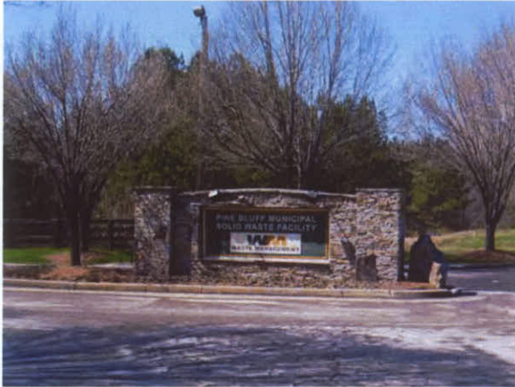
Figure 5-1: Entrance to Pine Bluff Landfill
