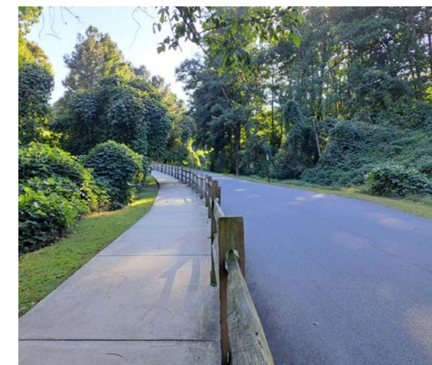
Sidepath Along Olde Rope Mill Park Road in Woodstock
