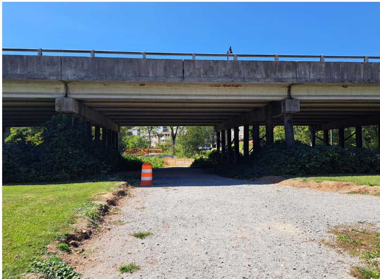
Extension of Etowah River Trail Near Waleska Street in Canton Under Construction in Fall 2023
