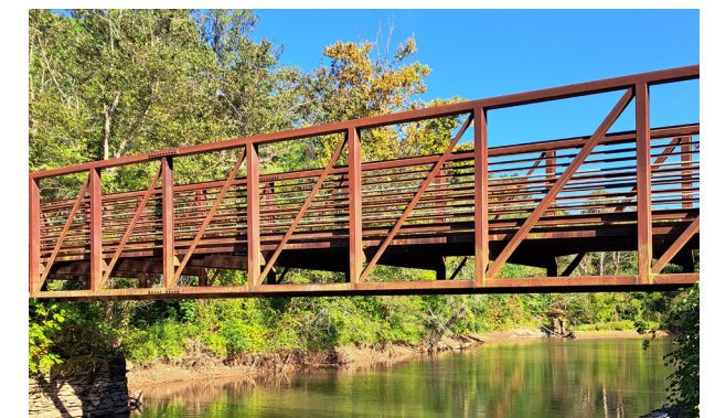
Pedestrian Bridge Over the Little River in Woodstock's Olde Rope Mill Park
