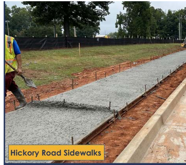
Hickory Road Sidewalks Construction - Cherokee SPLOST Program
